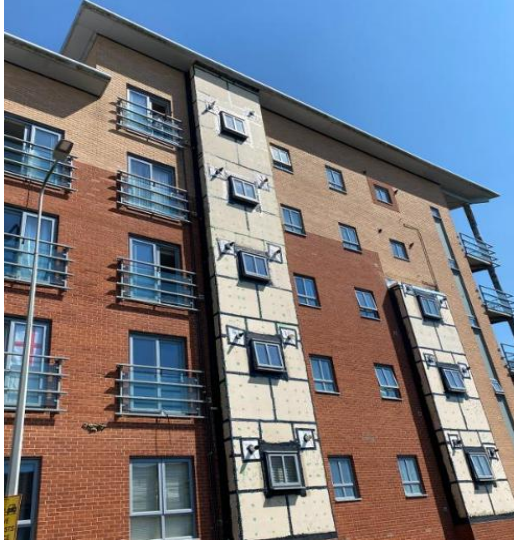
A photo showing Panels stripped and CP Board installed
