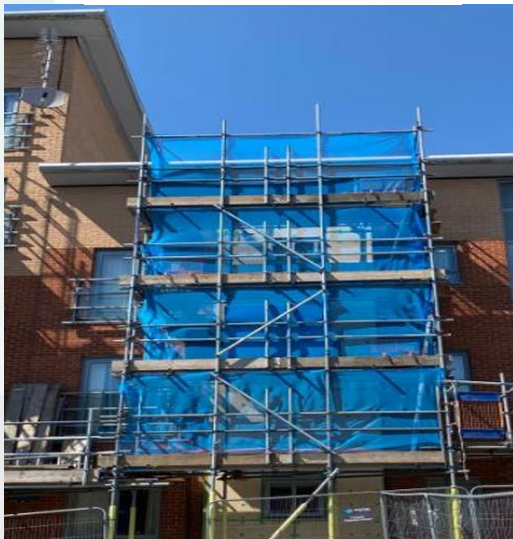
A photo showing Progression on Elevation B2
