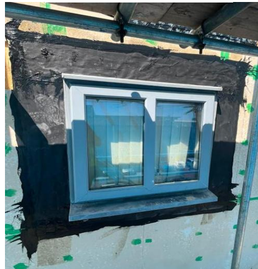
A photo showing CP board and EPDM being installed
